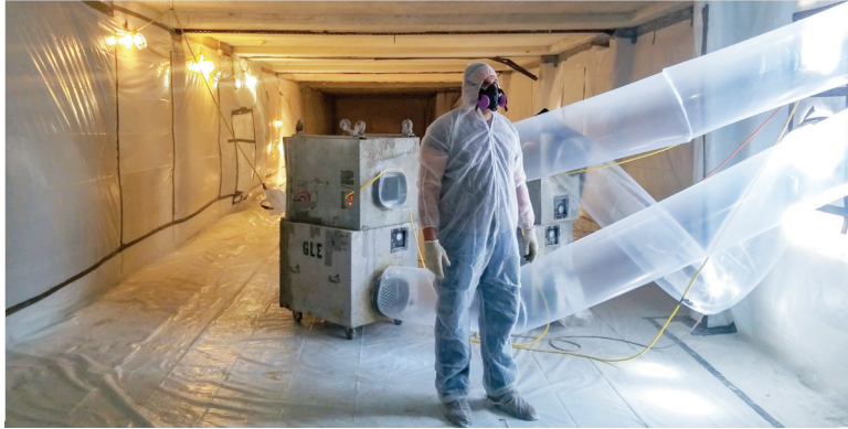
Iris Environmental Laboratories specializes in mold and asbestos laboratory analysis and field inspections. Here is one of Iris' inspectors performing air monitoring.
